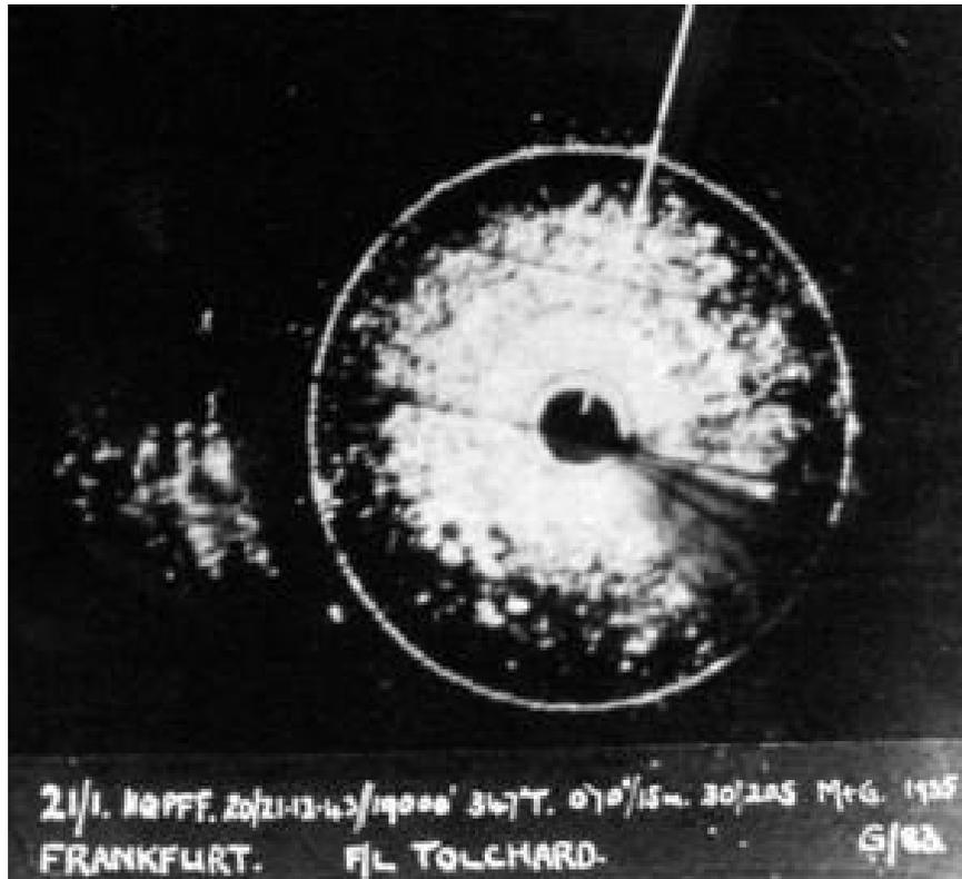
Figure 8: A transparency that could be placed over an H2S display to aid navigation, with annotations. [26]
