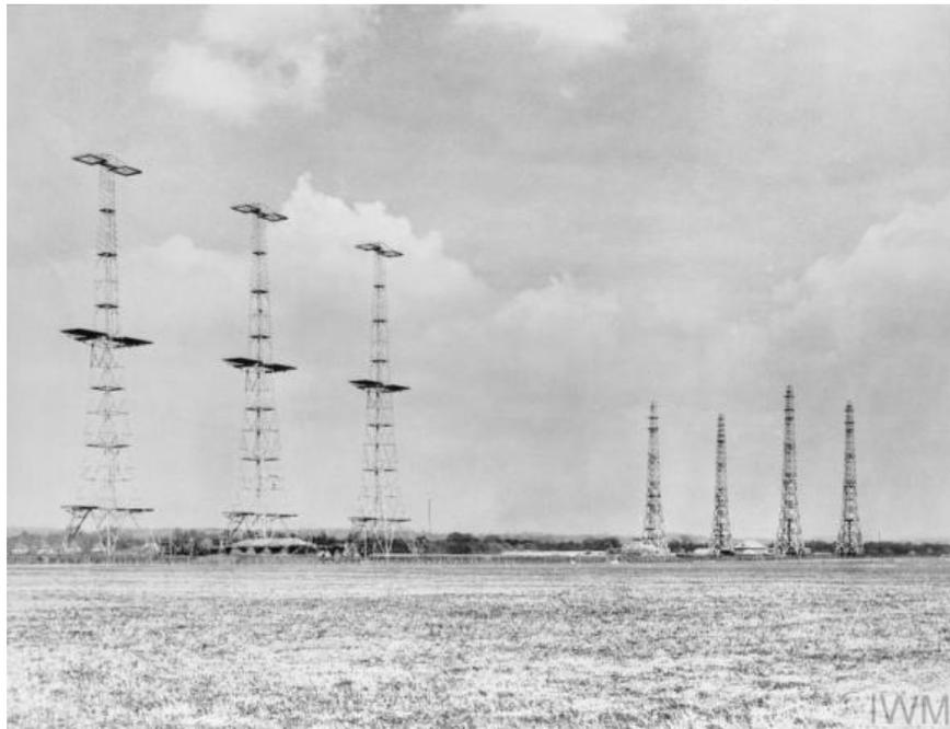
(b) A photograph of a Chain Home station in Poling, Sussex. Note the three large towers on the left of the image are transmitters and the four smaller (240') towers at the right of the image are the receive antennas, with the receiver station in the middle. [17]
