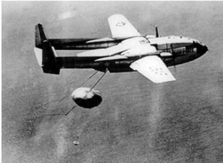
**Figure 16 – First Generation MAR Capture Using a C119 [20]**
